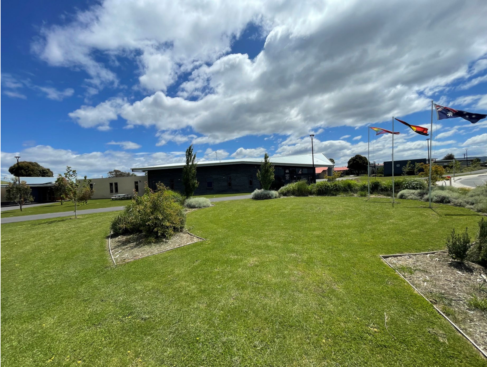
Circular Garden / lawn area (looking toward the Administration building)
