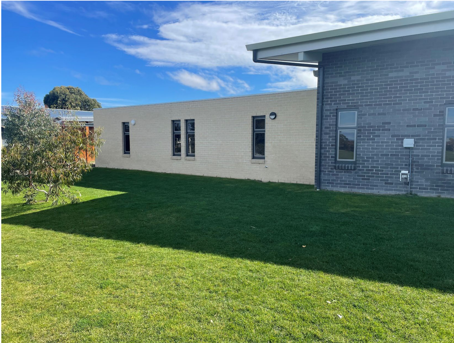
wall of Administration building (extended)
